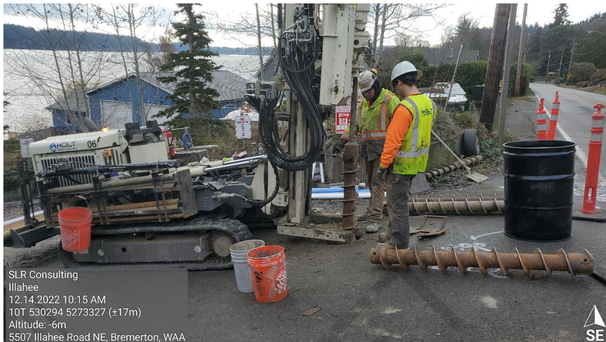
Photo 2 - Installation of MW-8
