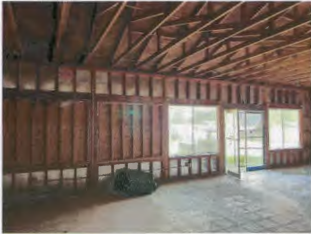
Interior north wall:
