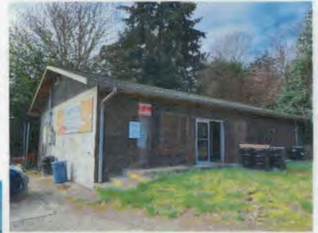
Existing Illahee store, exterior north and east walls:
