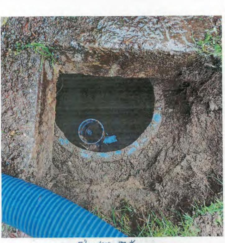
FibergLASS TANK Inlet OF SEPTIC TANK 1200 GALLONS.
